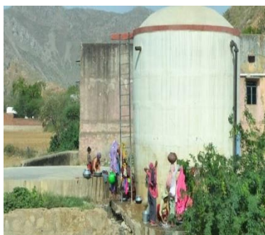
Figure 24 Dungarpur Water Tank
