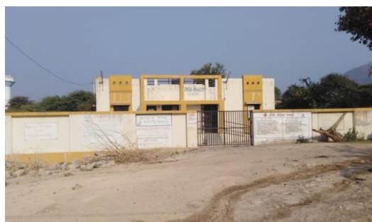
Figure 35 Existing Situation Sub Center
