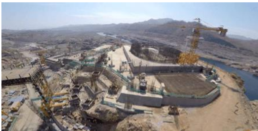
Construction of raft foundation of Statue of Unity
